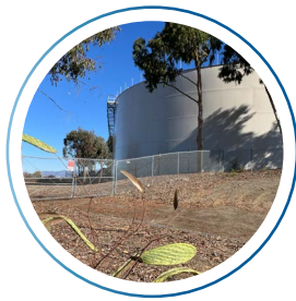
12 Closed Steel Tanks
